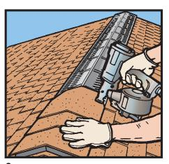
**6.** Center shingle cap on vent and nail along "NAIL HERE" guideline. Continue applying caps until all vent is covered with ridge caps. Do not overdrive nails. Nail head should be flush with top of shingle, without indenting it. Pre-forming caps in cold weather helps avoid cracking.
